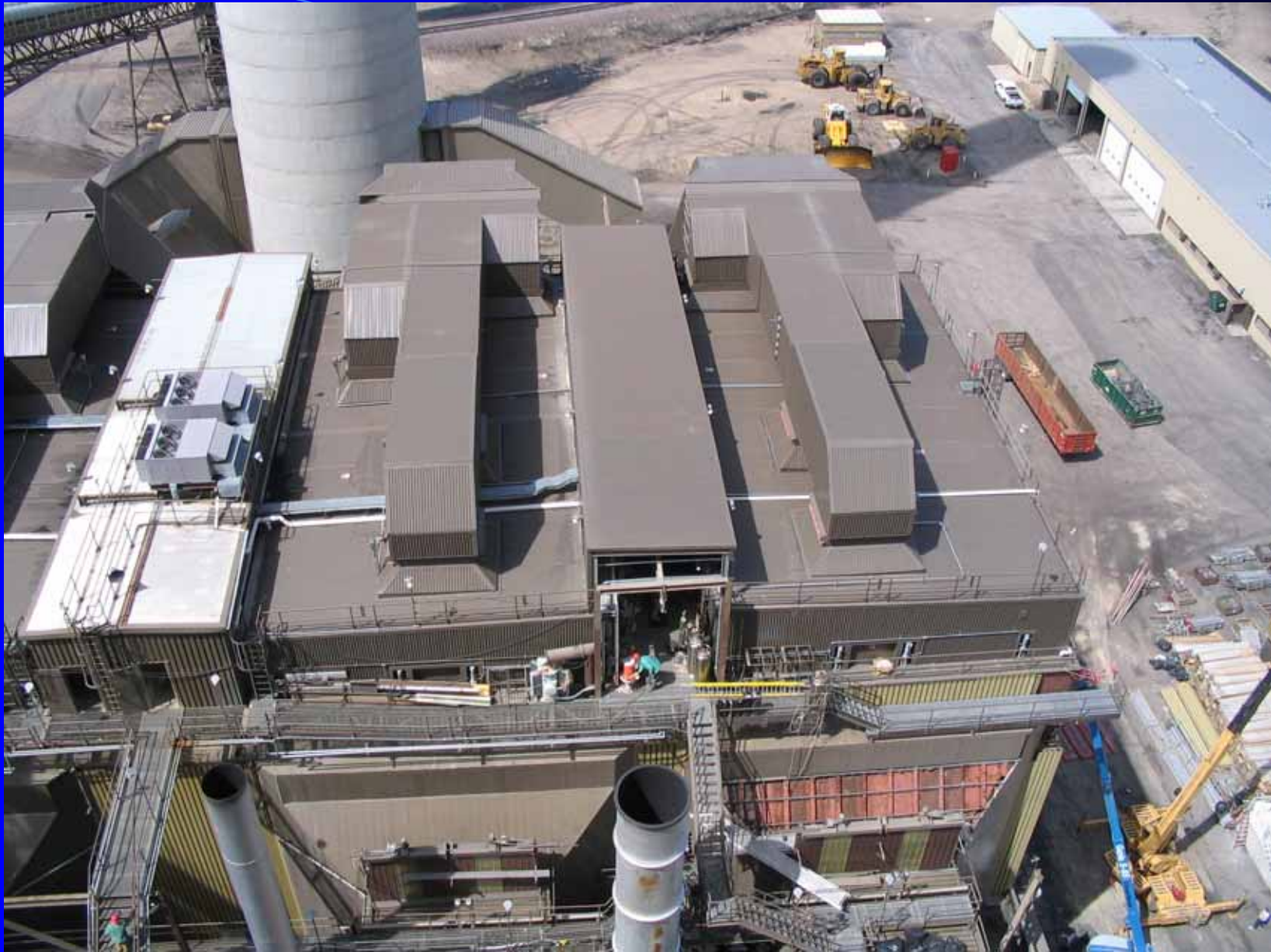
Big Stone Two North Chambers
